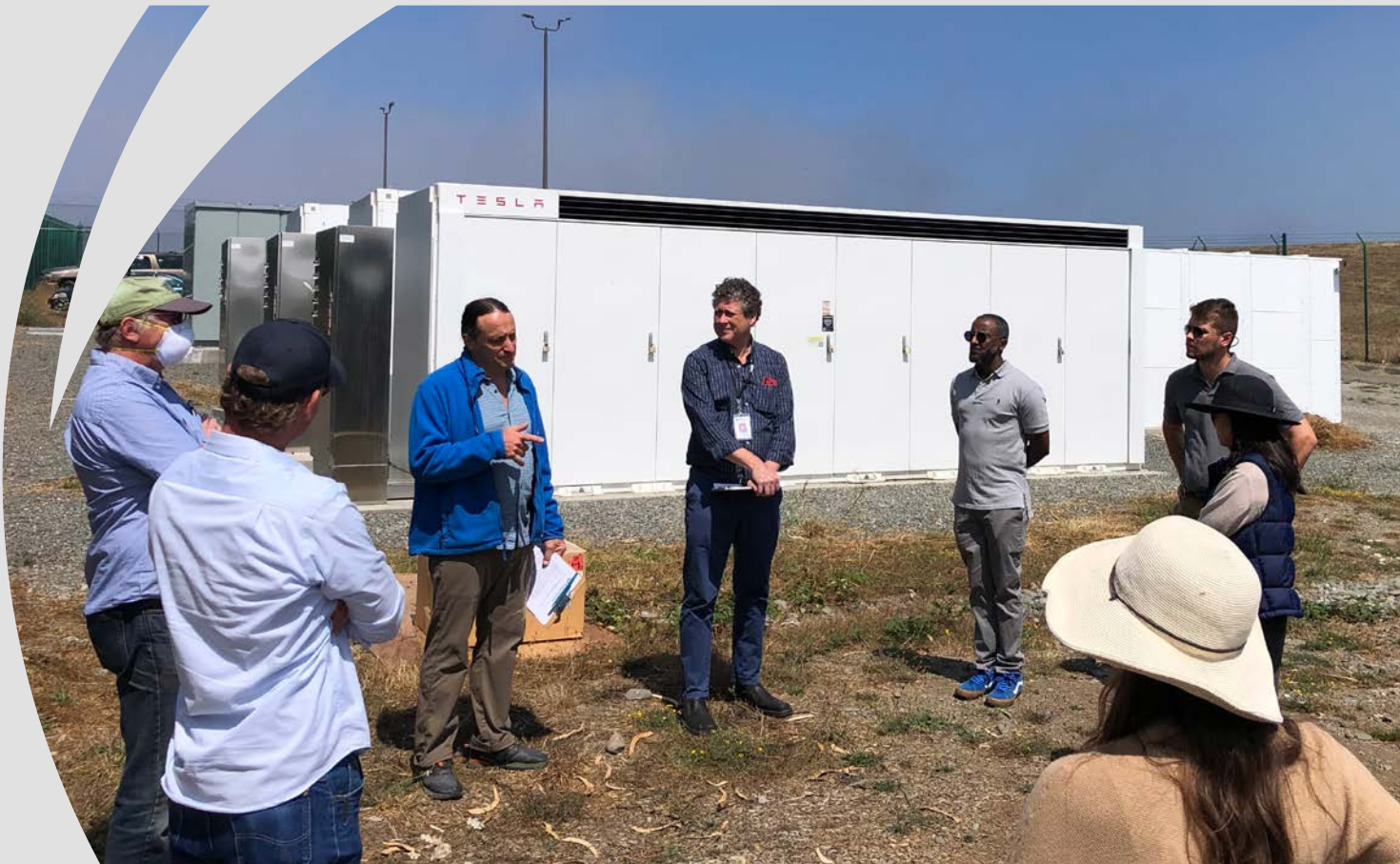
Photo: Public Advocates Office staff at Redwood Coast Airport Microgrid.
