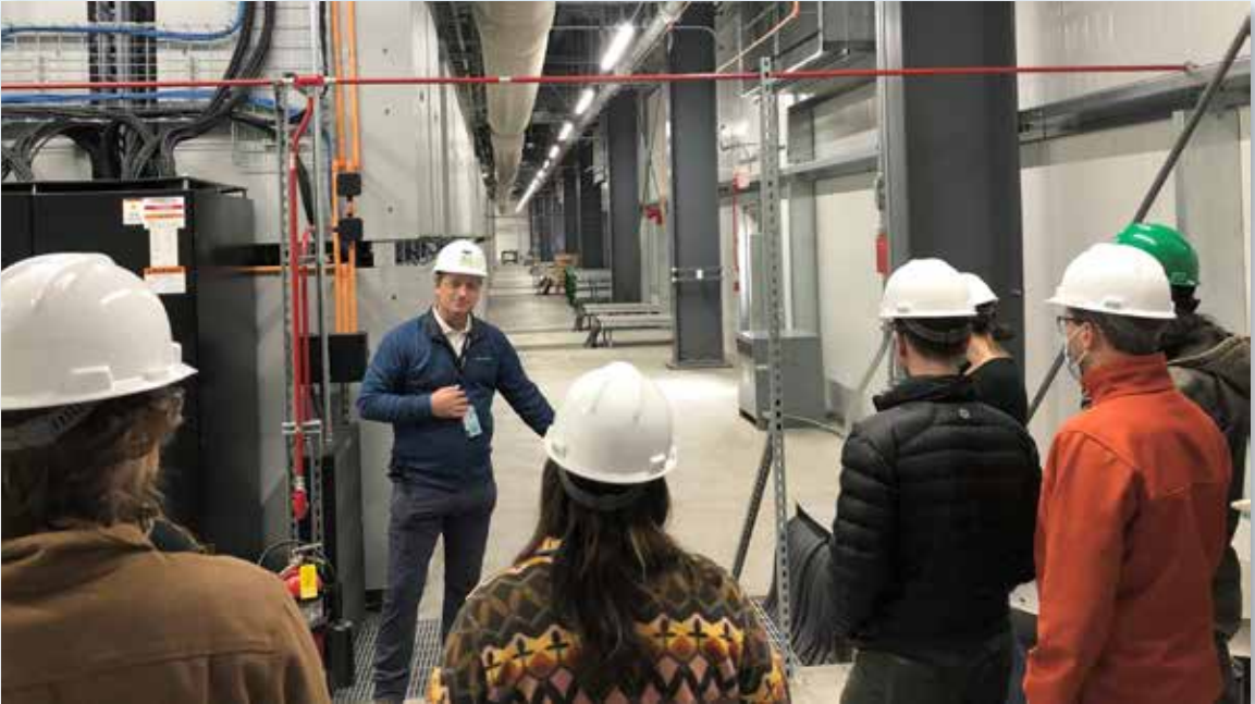
Tour of Moss Landing Power Plant.
