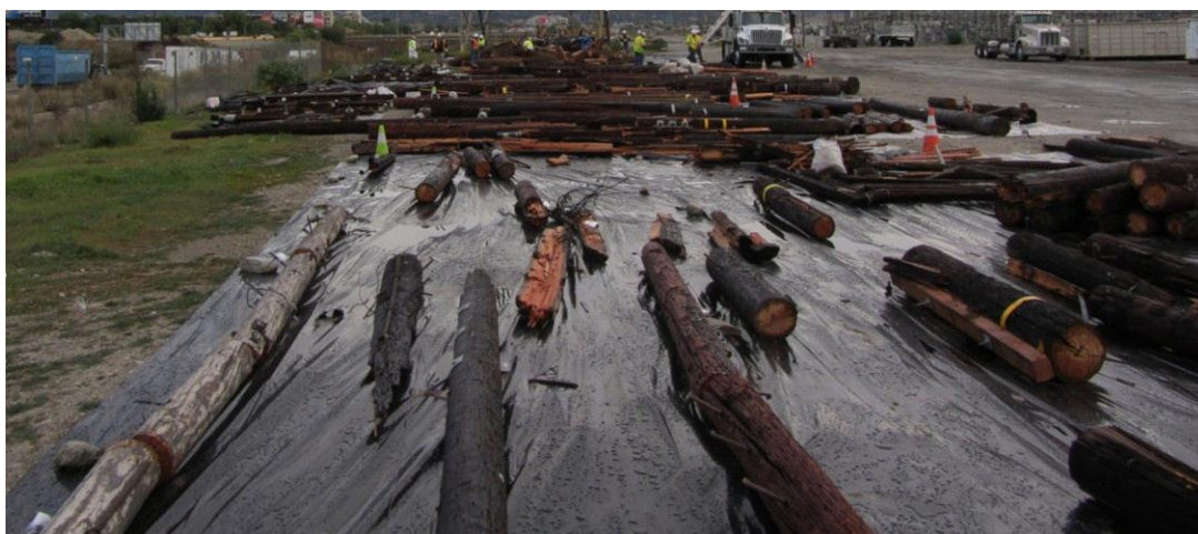
Figure 4 Portion of pole segments at Rio Hondo substation
